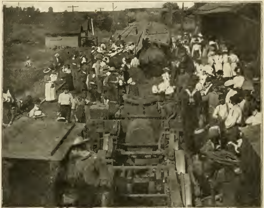
EXPLODED BOILER THROWN SEVENTY FEET AHEAD ON TRACK.
